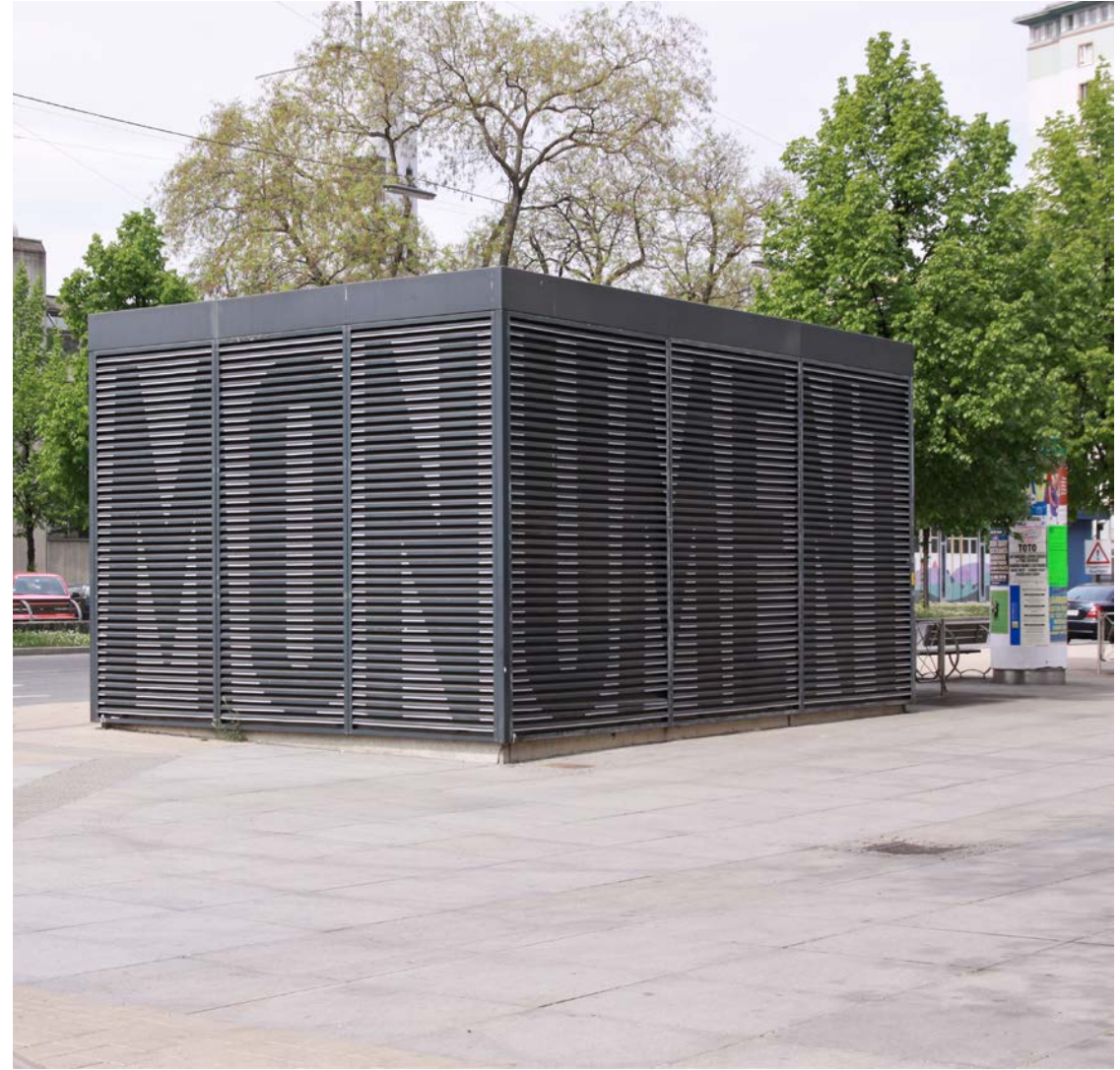
noneventmonument IV, 2010 - ? unannounced intervention, tape on existing transformer station Lendplatz, Graz
